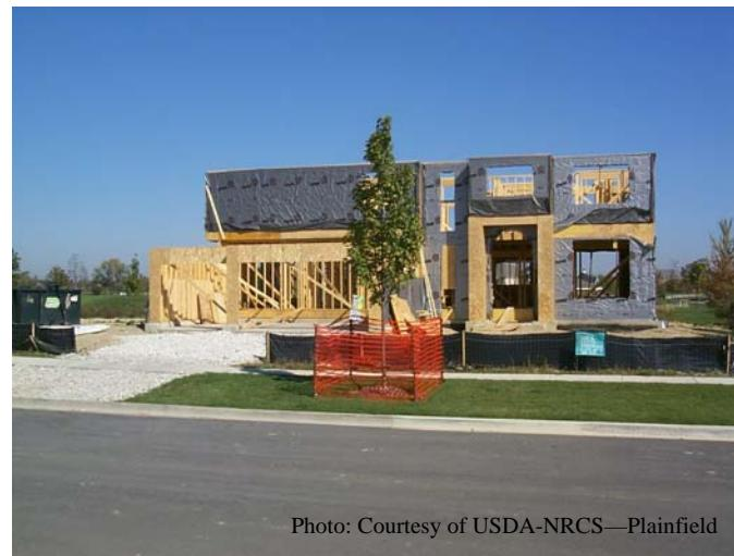
Erosion control is important even for home sites of an acre or less. The materials needed are easy to find and relatively inexpensive - straw, silt fence, stakes, gravel, plastic tubes, and grass seed. Putting these materials to use is a straightforward process. Only a few controls are needed on most sites:
