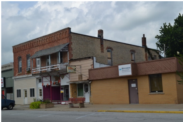
FIGURE 336. 147 West Station Street. Note the use of brick masonry for the street facade but limestone masonry for the party wall at the side.
